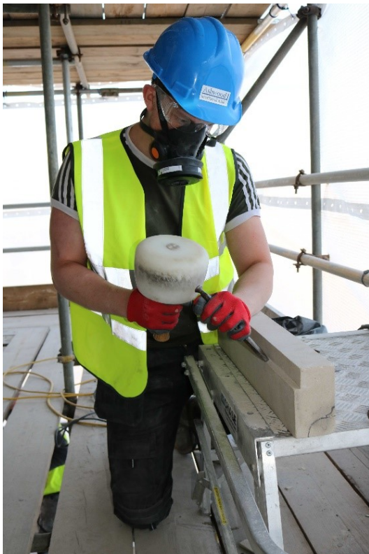
Lewis Docker, Apprentice stone mason shaping a stone edging before it is fitted into place.
