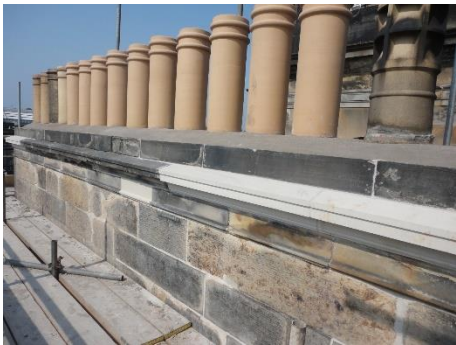
Stonework repairs to deteriorated chimney
