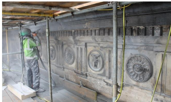
Low pressure soft abrasive cleaning
