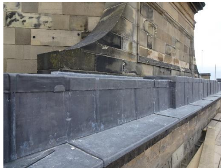
New lead upstand flashings
