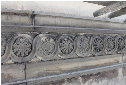
Section of cleaned decorative moulding
