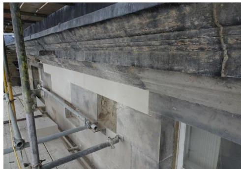
New lead cornice flashings and replacement stone
