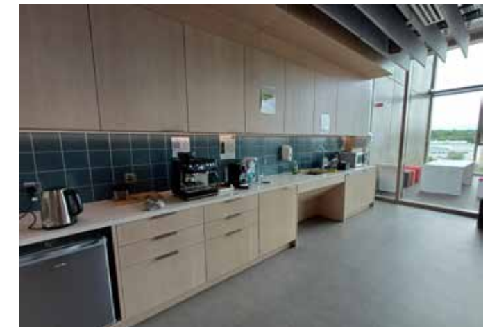
Pantry area in Usher Institute with a counter top at 850mm AFFL and open space under sink
