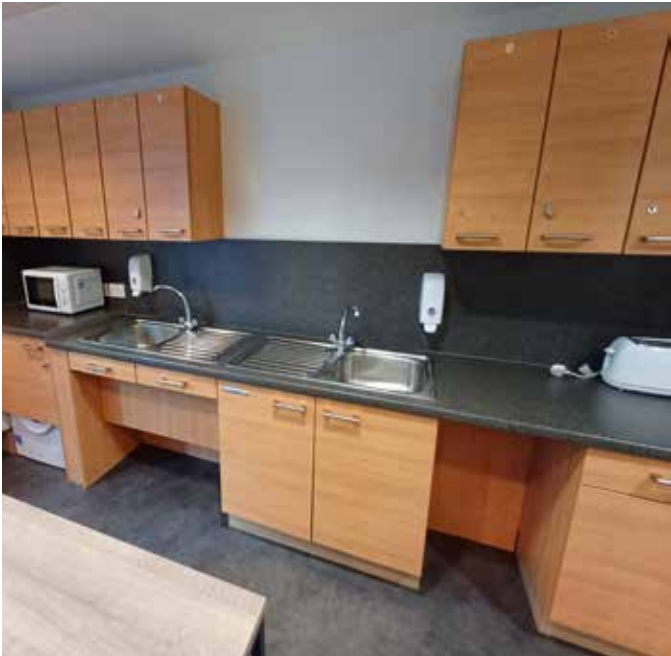
Accessible shared pantry, Chancellors Court, Pollock Halls of Residence. Note lowered counter at 850mm AFFL and two sinks, one open below. An improvement would be to have the tap to the side of the sink rather than at the back
