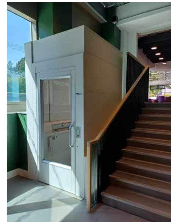
Enclosed platform lift adjacent to stair, connecting the Nucleus Building to adjacent Noreen & Kenneth Murray Library
